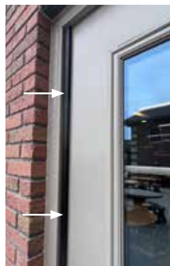
CONTINUOUS HINGE - CLOSED
