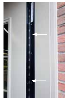
CONTINUOUS HINGE - OPEN
