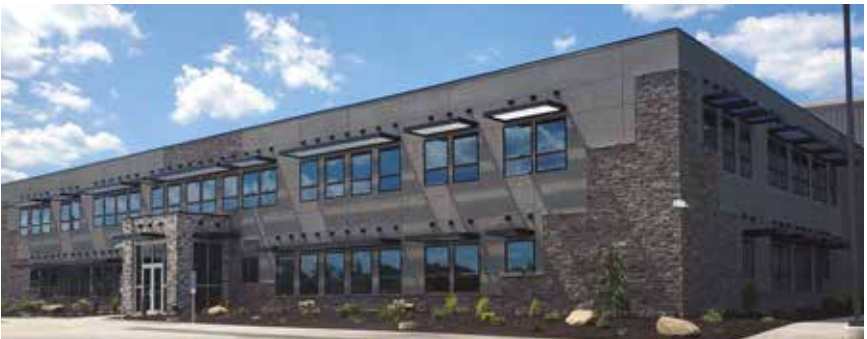
28,500 square feet of office space was completed at the Strasburg facility in July of 2020.
