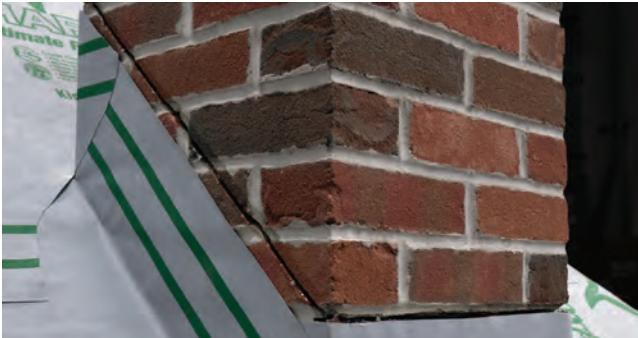
Fig. 31.1 - Chimney cut for Sidewall and Apron
