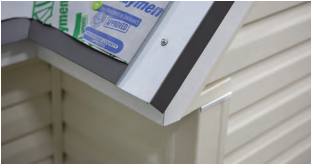
Fig. 13.1 - Outside corner piece installed
