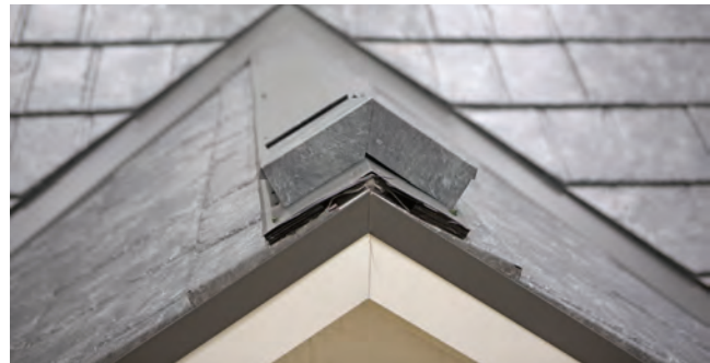
Fig. 38.2 - First Ridge Cap ready to install
