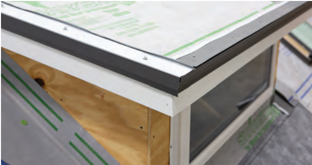
Fig. 15.1 - Outside corner piece installed
