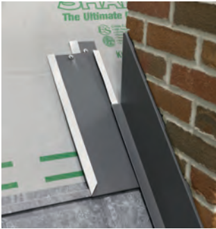
Fig. 29.1 - 6" Underpan installed at the top of a chimney
