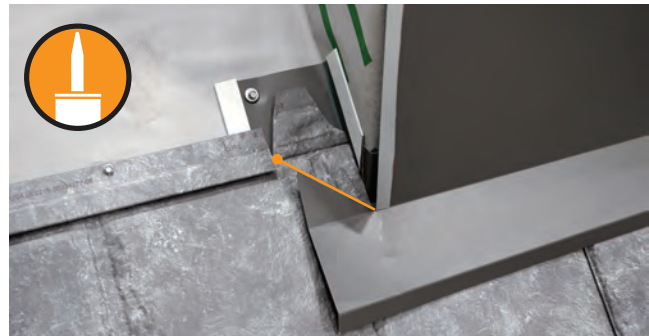
Fig. 32.1 - Top lock cut and bent open
