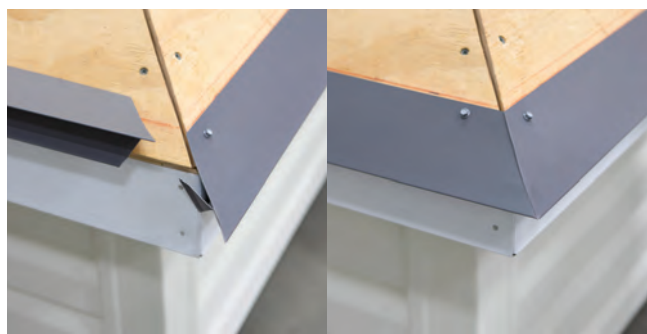
Fig. 12.4 - Second outside corner piece installed
