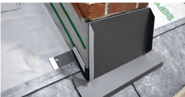
Fig. 31.4 - Apron flashing installed
