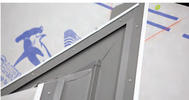
Fig. 17.4 - Valley flashings installed at ridge
