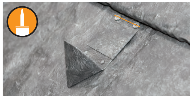
Fig. 39.3 - Standard diverter installed
