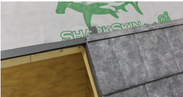
Fig. 27.3 - Panels installed to Eave Starter
