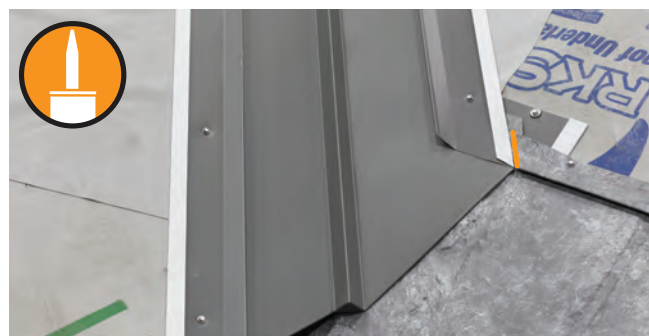
Fig. 18.4 - Valley flashing installed in floating valley
