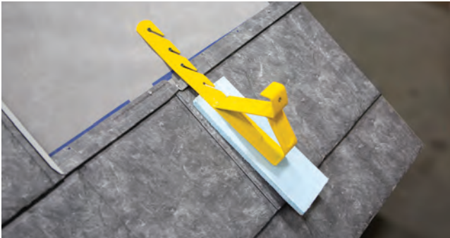
Fig. 9.1 - Roof jack installed
