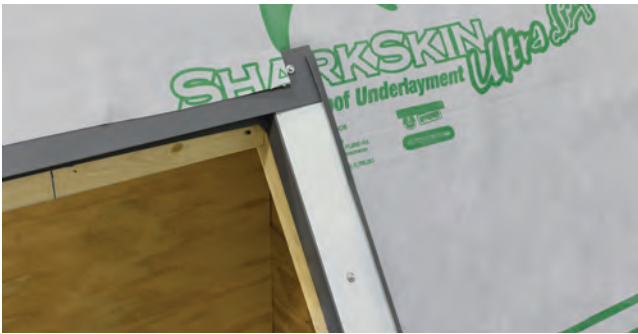
Fig. 27.1 - Eave Starter and Rake Trims installed
