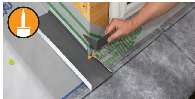
Fig. 28.2 - Underpan installed
