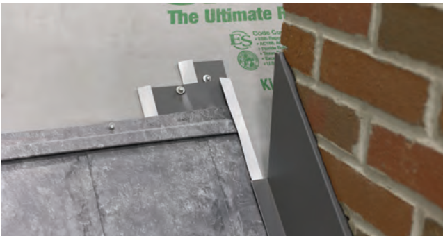
Fig. 33.1 - Panels installed beyond top of chimney
