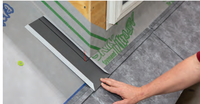
Fig. 28.1 - Underpan marked
