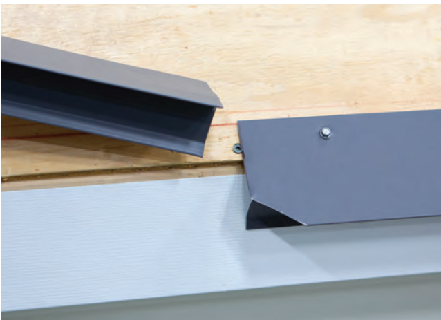
Fig. 11.2 - Overlap pieces cut and ready to install
