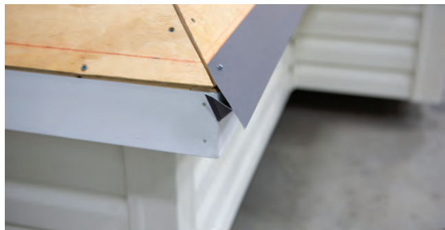
Fig. 12.3 - First outside corner piece installed
