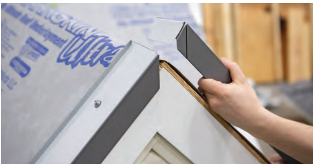
Fig. 13.3 - Plumb cut and next piece ready for install
