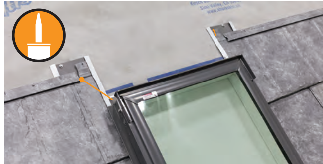
Fig. 36.1 - Panels installed and top lock opened
