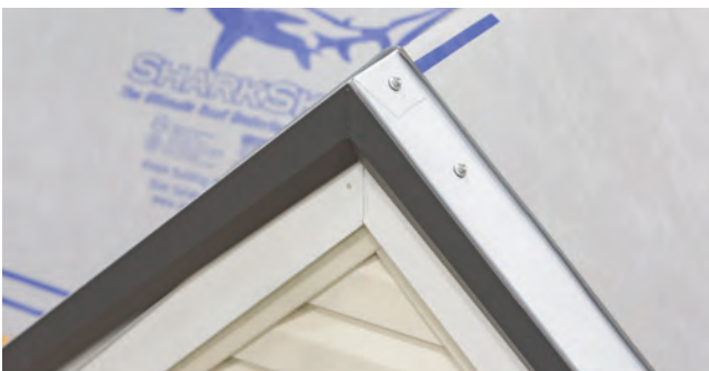
Fig. 15.4 - Second piece at peak installed
