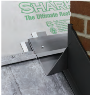
Fig. 29.1 - 6" Underpan installed at the top of a chimney
