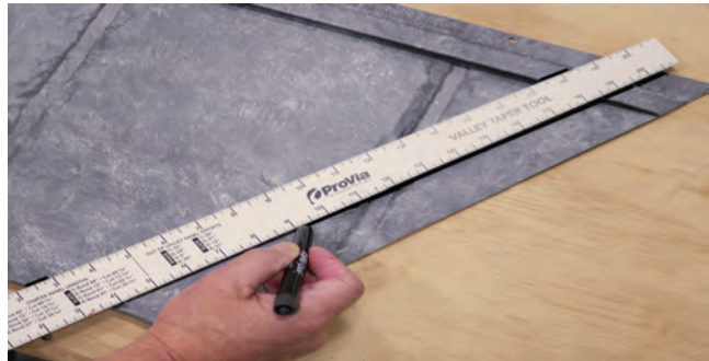
Fig. 24.2 - Mark cut line
