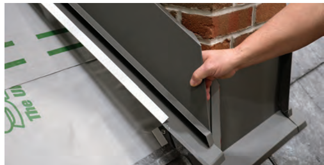
Fig. 32.2 - Sidewall ready to install
