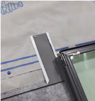
Fig. 29.2 - 6" Underpan installed at the top of a skylight
