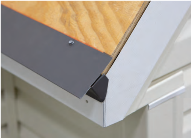
Fig. 11.1 - Outside corner piece installed
