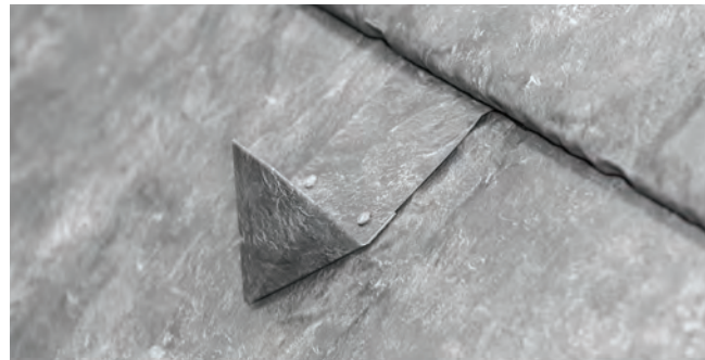
Fig. 39.2 - Panels installed over ProGrip diverter
