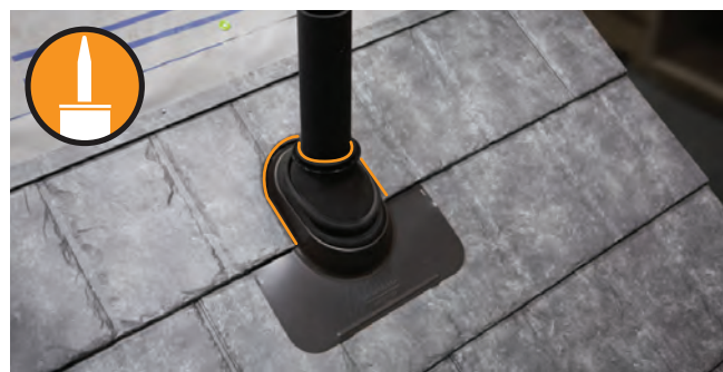
Fig. 30.4 - Panels installed around pipe flashing
