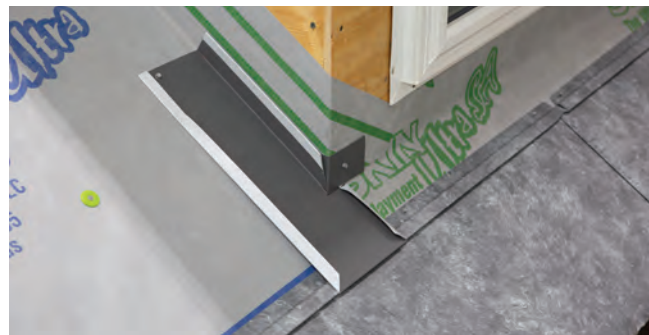
Fig. 28.3 - Underpan and corner shield installed
