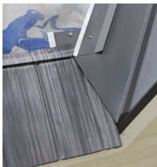
Fig. 29.4 - 6" Underpan installed at an eave to rake valley
