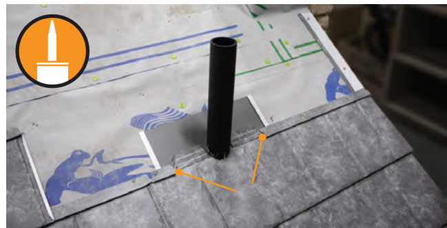
Fig. 30.2 - Panels installed around vent pipe
