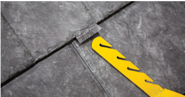
Fig. 9.3 - Roof jack removed
