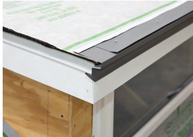
Fig. 14.1 - Outside corner piece installed
