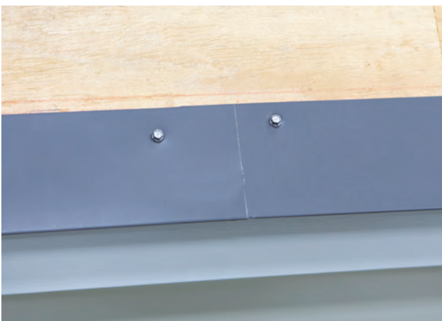
Fig. 11.3 - Overlap pieces installed
