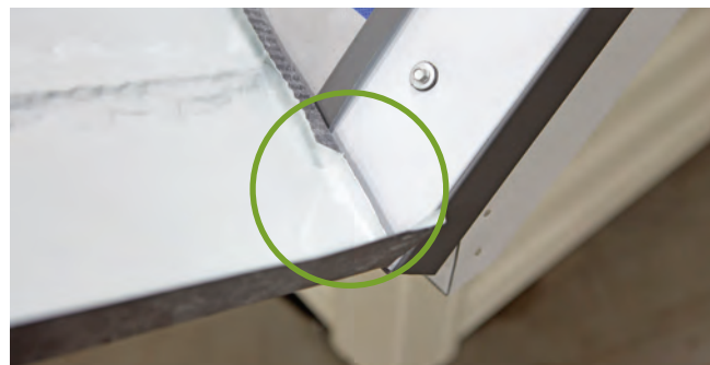
Fig. 20.4 - 2" drain slot
