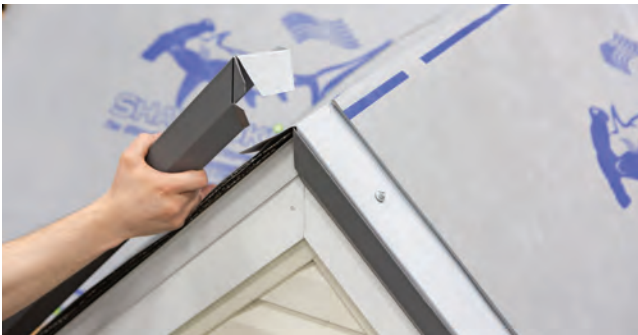
Fig. 15.3 - First piece at peak installed
