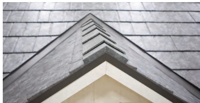
Fig. 38.4 - Ridge Cap installed
