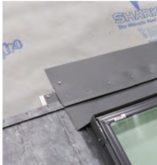
Fig. 29.2 - 6" Underpan installed at the top of a skylight
