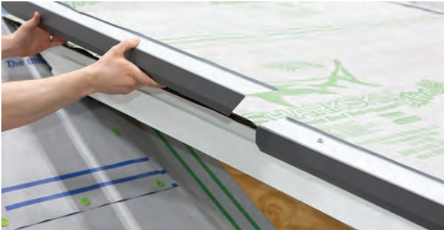
Fig. 15.2 - Overlap piece ready to install
