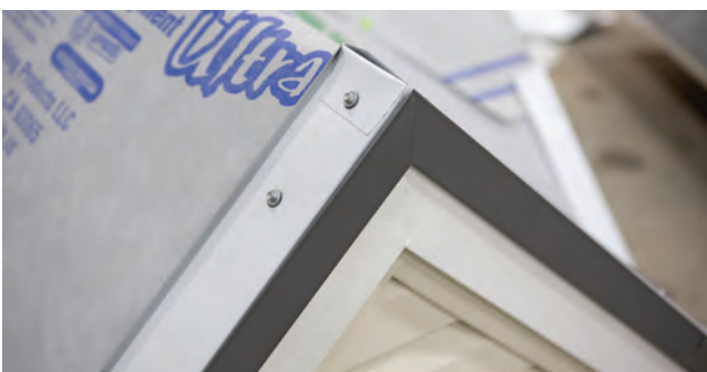
Fig. 13.4 - Second piece at peak installed
