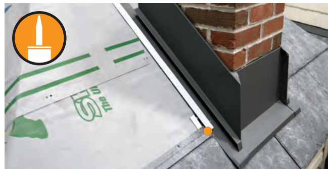
Fig. 32.3 - Sidewall installed at chimney
