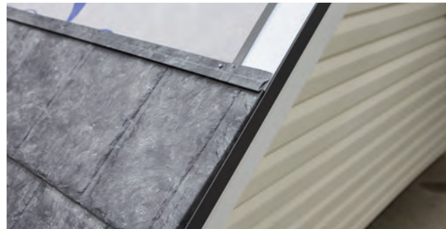
Fig. 20.3 - Panel installed into Rake Trim
