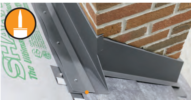
Fig. 33.4 - Backflash and Anchor Cleat installed
