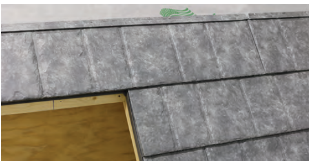
Fig. 27.4 - Installed short course
