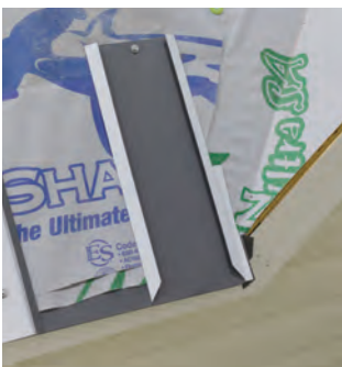
Fig. 29.4 - 6" Underpan installed at an eave to rake valley
