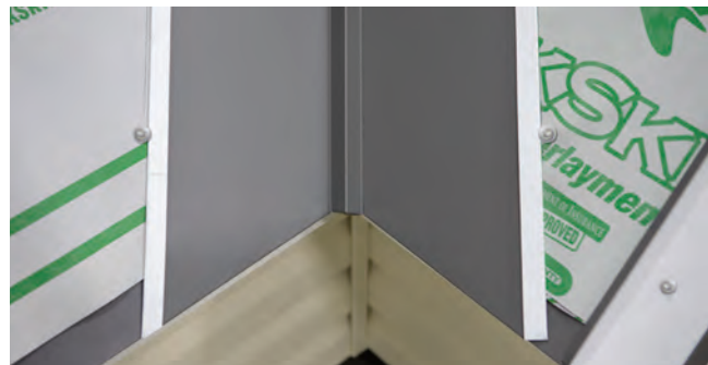
Fig. 16.3 - Valley flashing installed
