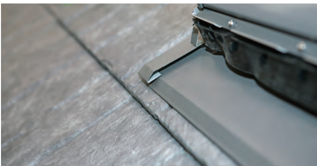
Fig. 35.4 - Open hem at bottom of sidewall
