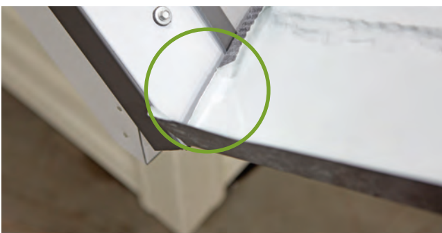
Fig. 19.4 - 2" drain slot in the first piece
