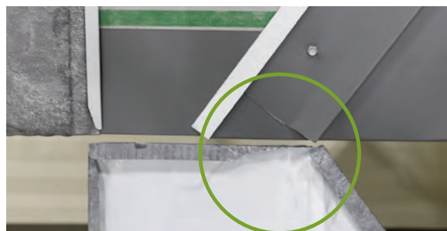
Fig. 22.4 - 2" drain slot in first panel
