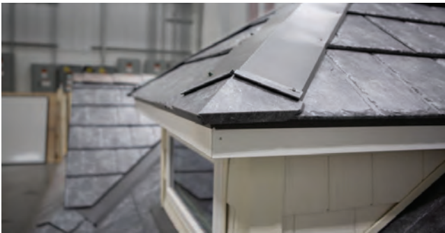
Fig. 37.3 - First Ridge/Hip Cap installed
