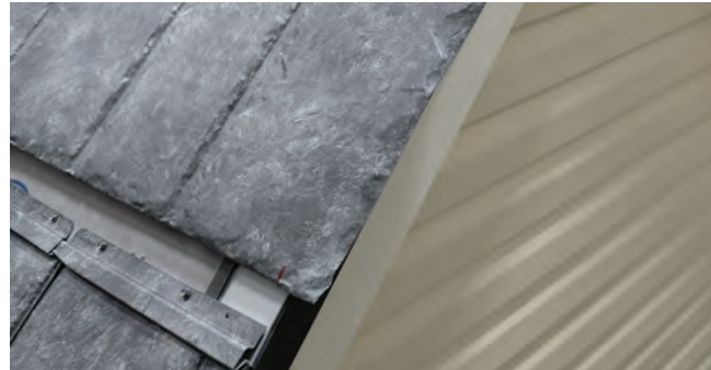
Fig. 20.1 - Panel cut and ready to fold
