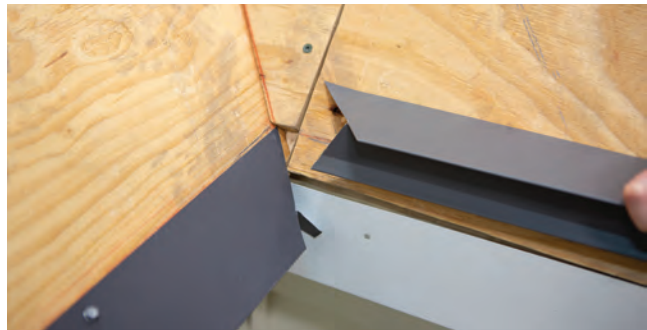
Fig. 12.2 - Second inside corner piece ready to install
