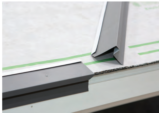
Fig. 14.2- Overlap pieces cut and ready to install
