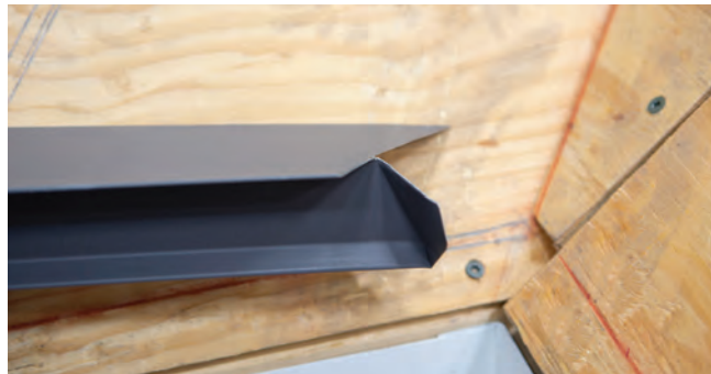
Fig. 12.1 - First inside corner piece ready to install
