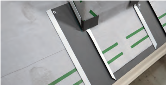
Fig. 31.2 - Underpan installed at chimney
