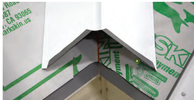
Fig. 16.2 - Valley flashing ready to install
