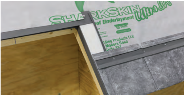
Fig. 27.2 - First course of panels and Anchor Cleat installed
