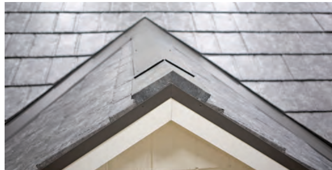
Fig. 38.3 - First Ridge Cap installed
