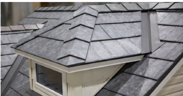
Fig. 37.4 - Ridge/Hip Cap installed
