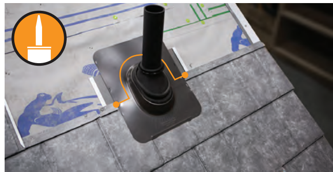
Fig. 30.3 - Pipe flashing installed over panels
