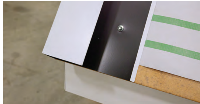
Fig. 12.1 - C-Closure installed on the rake
