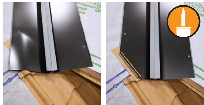
Fig. 16.2 - Valley Closures installed
