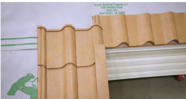
Fig. 21.3 - Panels with top lock trimmed
