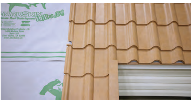
Fig. 21.4 - Panels installed above the short course
