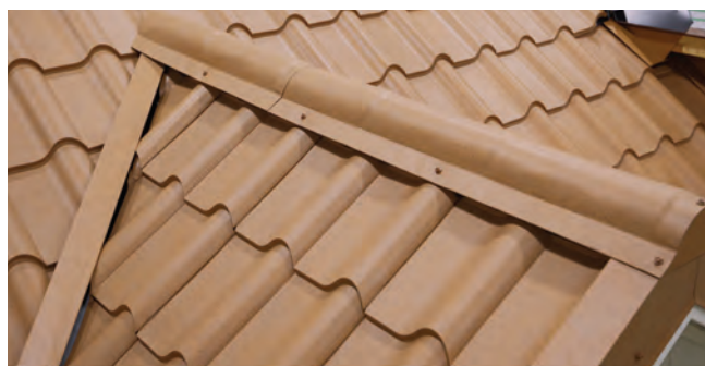
Fig. 30.4 - Ridge/Hip Cap installed
