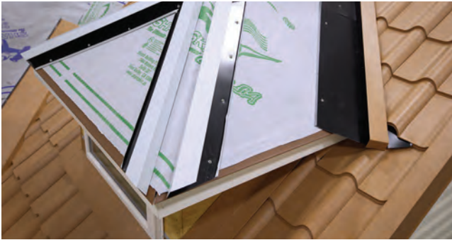
Fig. 29.1 - C-Closures installed at hip
