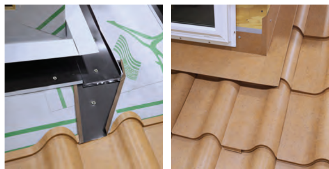
Fig. 22.4 - C-Closure and bottom lock on panel opened
