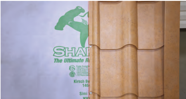
Fig. 19.1 - Panel installed at Rake with vertical chalk line
