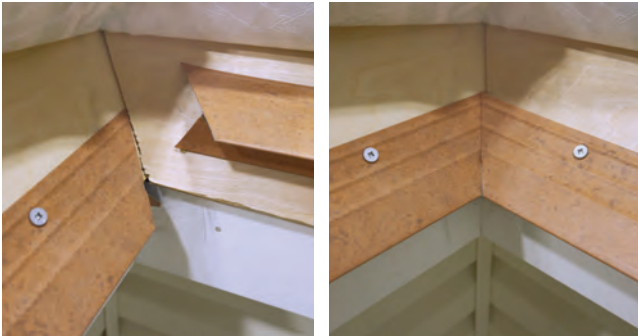
Fig. 11.2 - Remaining piece cut and installed
