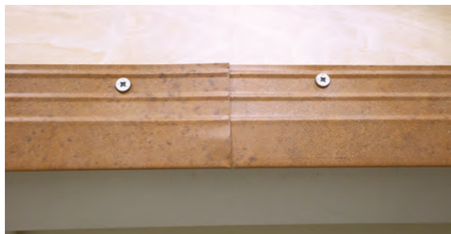
Fig. 10.4 - Overlap piece installed
