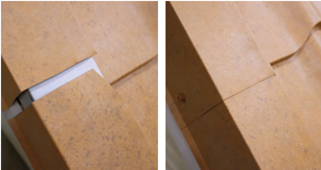
Fig. 13.2 - Overlapping Rake installed
