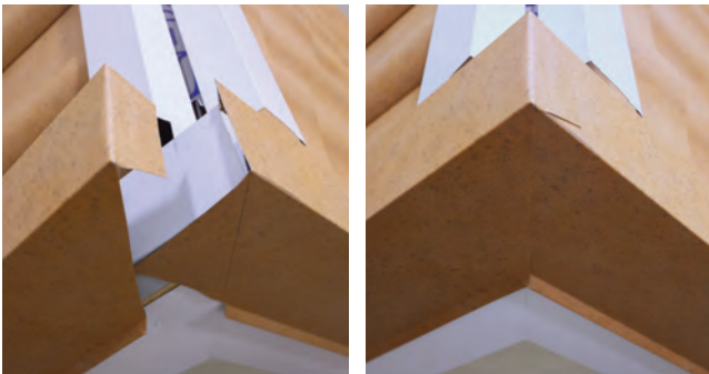
Fig. 13.3 - Rake installed at ridge peak
