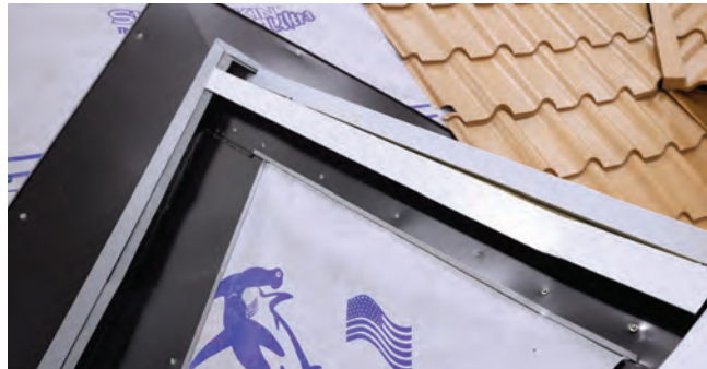
Fig. 30.1 - C-Closures installed at ridge
