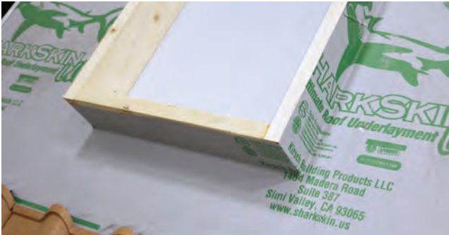
Fig. 27.1 - Underlayment installed around skylight
