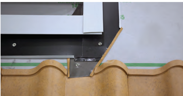
Fig. 27.4 - Weep trim installed at bottom corner
