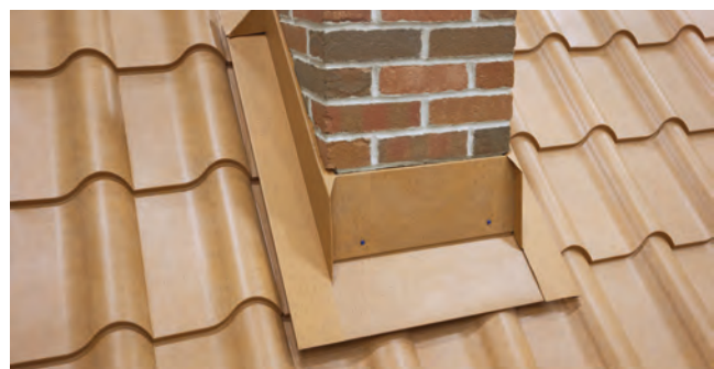
Fig. 26.4 - Panels installed around the chimney
