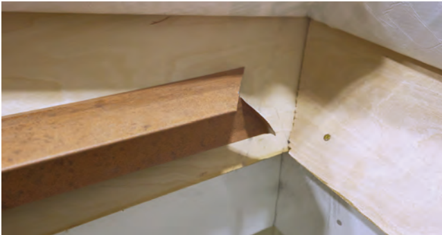
Fig. 11.1 - First inside corner piece ready to install
