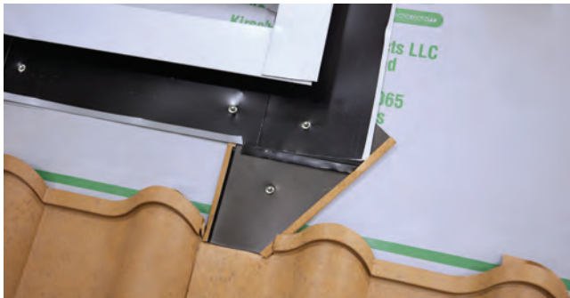
Fig. 25.3 - Weep trim installed at bottom corners
