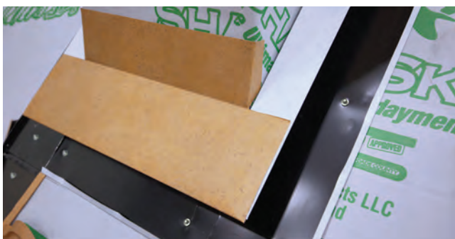
Fig. 25.4 - Apron installed at bottom of chimney
