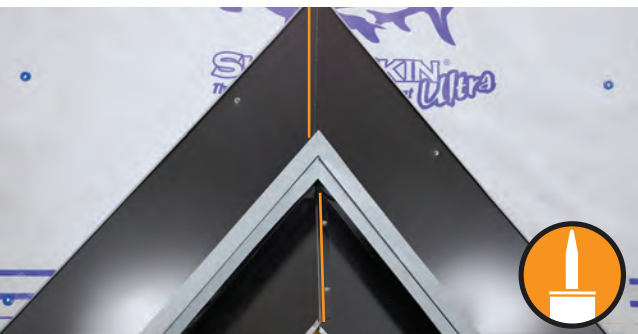
Fig. 15.4 - Valley Closures installed at ridge
