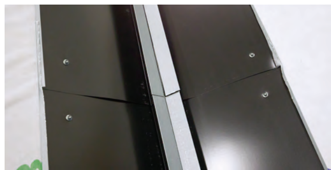
Fig. 14.4 - Overlap piece installed
