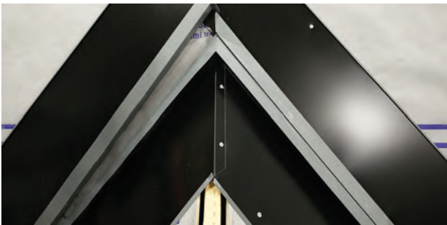
Fig. 15.2 - Second pieces ready to install
