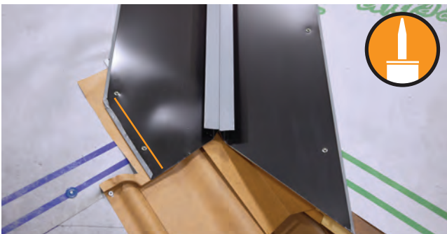
Fig. 17.3 - Water stop formed on Valley Closure
