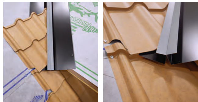
Fig. 16.3 - Panel installed into the Valley Closure
