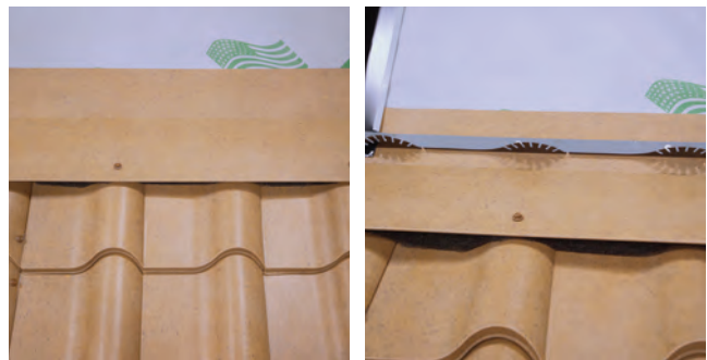
Fig. 20.2 - Transition trim installed at pitch change
