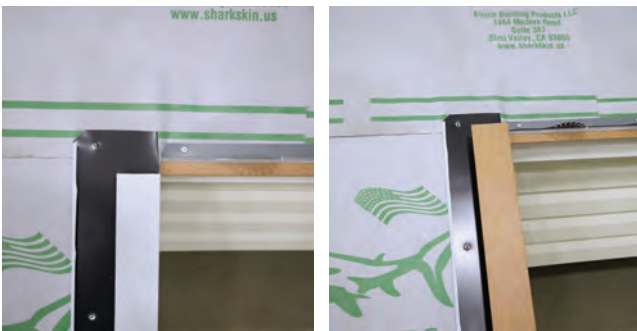
Fig. 21.2 - C-closure, Rake, and Bird Stop installed
