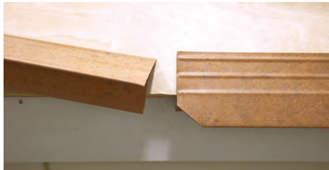
Fig. 10.3 - 1" angle cut and overlap piece ready to install
