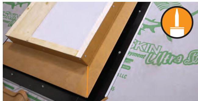
Fig. 28.2 - Sidewall installed on the sides of skylight
