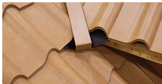
Fig. 16.4 - Panels and Valley Closure Cap installed
