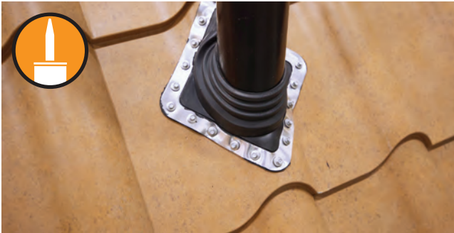
Fig. 23.2 - Vent pipe flashing fastened to panel
