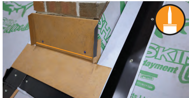
Fig. 26.1 - Counter-flashing installed
