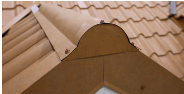
Fig. 30.2 - Ridge/Hip Cap and End Cap installed
