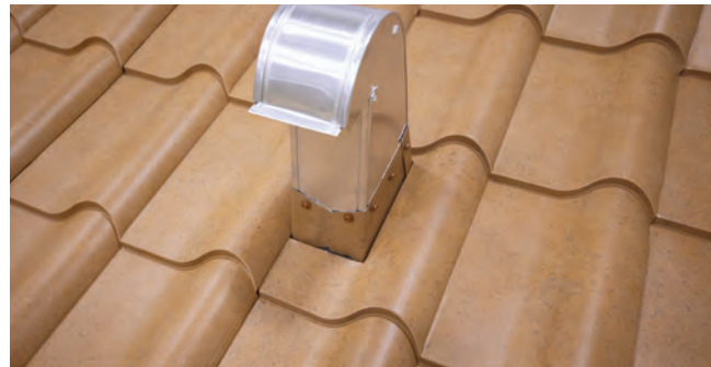
Fig. 24.3 - Panel installed around the pipe flashing
