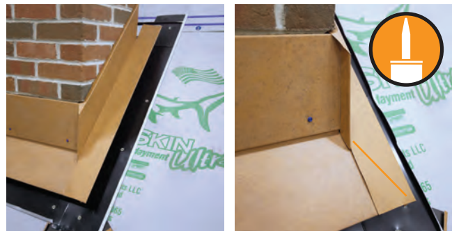
Fig. 26.2 - Sidewall installed
