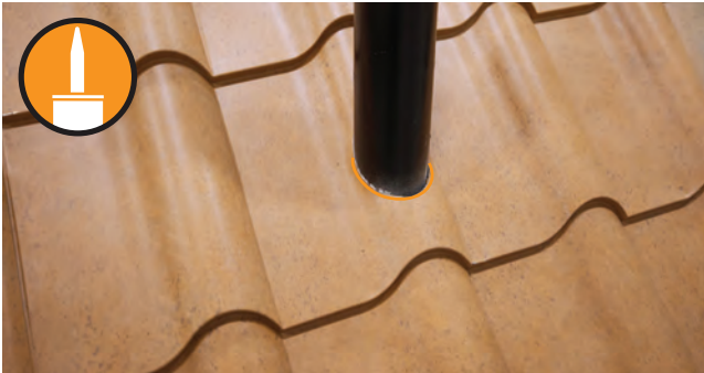
Fig. 23.1 - Panel installed around vent pipe
