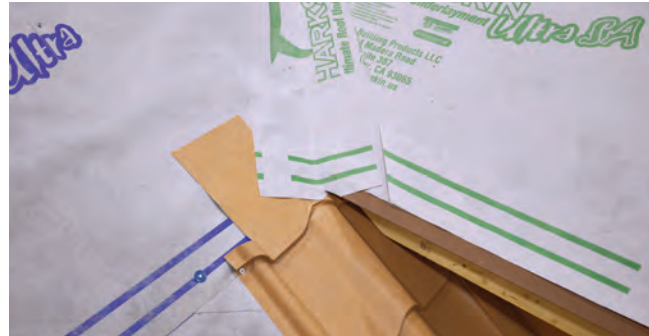
Fig. 16.1 - Panels installed before Valley Closure
