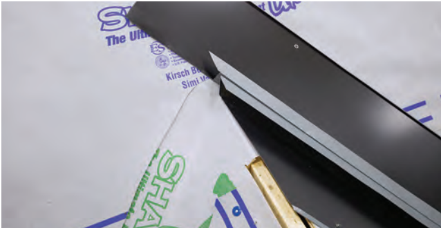
Fig. 15.1 - First pieces cut at the peak
