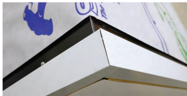
Fig. 12.4 - Second piece of C-Closure installed
