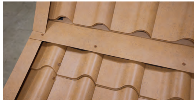
Fig. 20.3 - Panels installed above the pitch change
