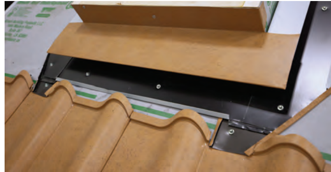
Fig. 28.1 - Apron installed at the bottom of skylight
