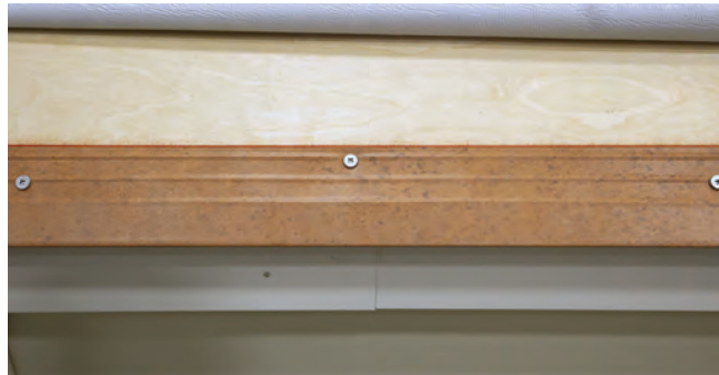
Fig. 10.1 - Eave Starter installed along chalk line
