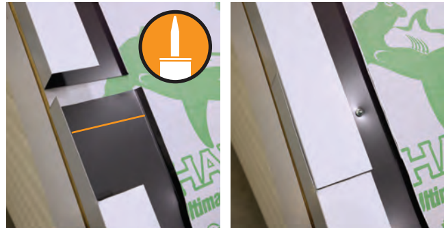
Fig. 12.2 - Overlapping C-Closure installed
