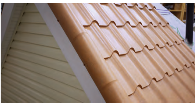
Fig. 13.4 - Ridge/Hip Cap installed at rake
