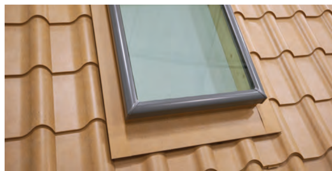
Fig. 28.4 - Panels installed around skylight
