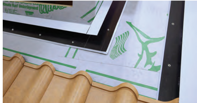
Fig. 22.1 - Panels installed below penetration point
