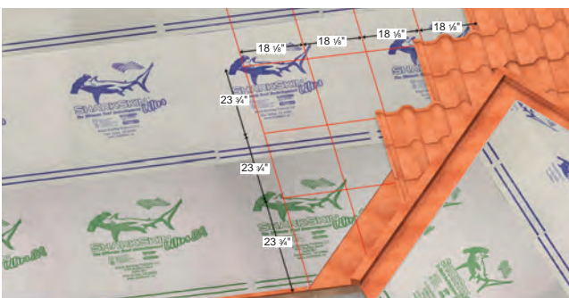
Fig. 19.4 - Panels installed at a dormer valley
